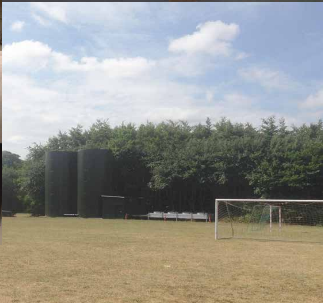
Below left: Machines cooling down smoke from the cremation, creating surplus hot water for district heating.
